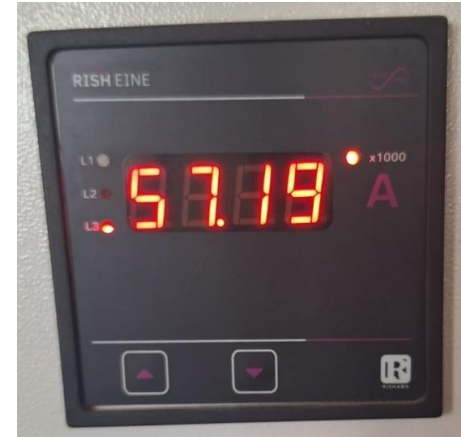
BOQ 31: Digital Ammeter for R,Y,B
