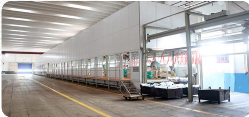
Automatic phosphate line
